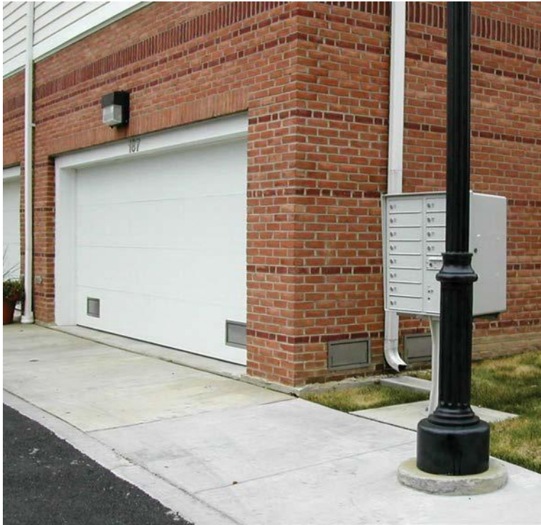
Figure 6: Engineered openings in garage doors
