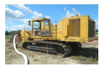
Figure 9 - Trench and Collector Pipe Installation (Courtesy of DeWind Trenching)
