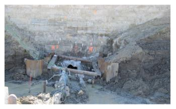
Figure 2 - Uncontrolled downstream seepage exiting with reservoir down to deadpool, rehabilitation of headworks, Lake Frances Dam, MT (Note pin boils near toe; the two wells were ineffective). (Courtesy of Montana Department of Natural Resources and Conservation)
