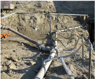
Figure 5 - Wellpoint system along trench excavation, Lake Frances Dam Outlet Works Rehabilitation, MT (Courtesy Montana Department of Natural Resources and Conservation)
