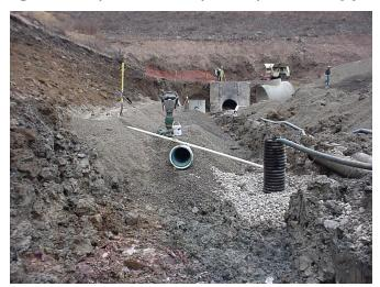
Figure 4 - Example of well-designed sump to collect both surface water and groundwater at Nevada Dam, MT (Courtesy Montana Department of Natural Resources and **Conservation**)
