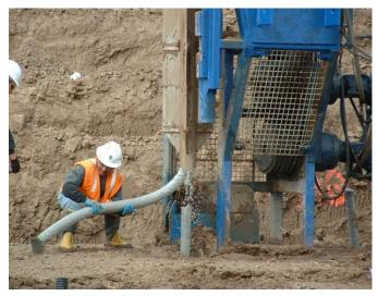
Figure 10 - Installation of Earthquake Drain by Hollow Mandrel Advanced with Vibratory Hammer (Courtesy of Hayward-Baker Inc.)
