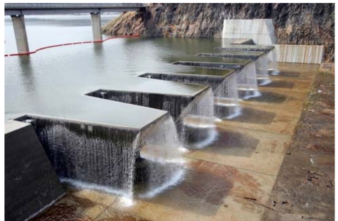
Figure 3. Labyrinth Weir Fusegate Spillway [6]
