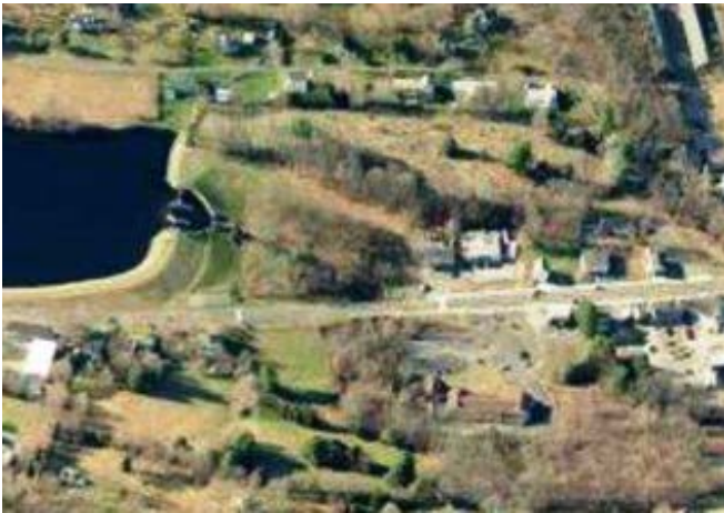
Figure 1. Downstream Development near the Dam Toe—a Hazard Creep Scenario [1]
