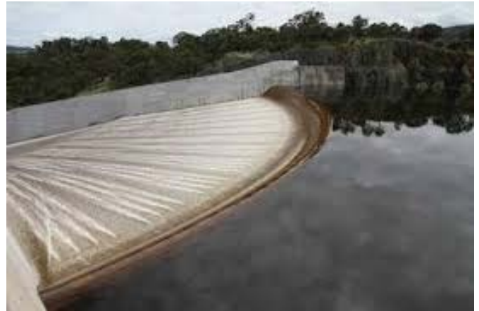
Figure 2. Arced Weir Spillway [5]
