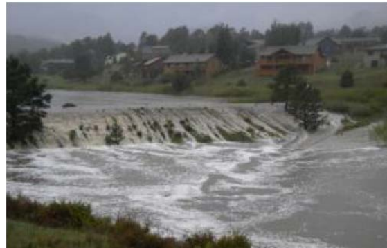
Figure 4. Overtopping of Earth Dam during a Rare Flood Event
