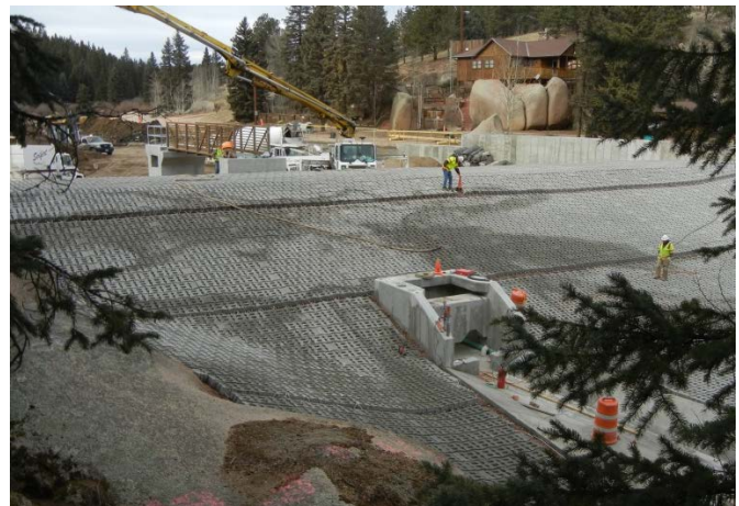
Figure 5. ACB Overtopping Protection
