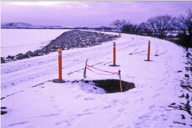
Figure 19. Sinkhole in crest of a dam in Montana that manifested after several years of undetected internal erosion into a damaged conduit [6]
