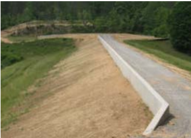
Figure 6. Dam Crest Raise with a Concrete Parapet Wall [9]
