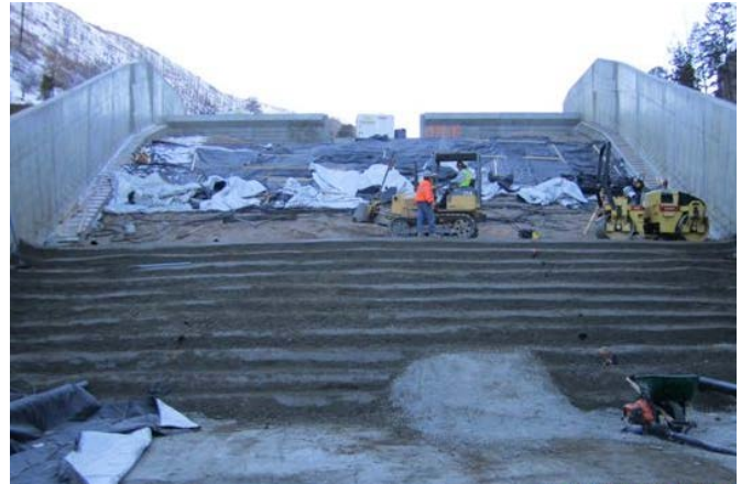
Figure 4. RCC Overtopping Protection Installation
