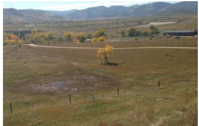
Figure 13. Seepage through Foundation Exiting at Downstream Toe of Earthen Dam
