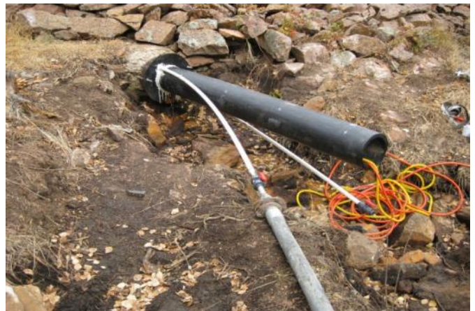
Photo 10: Grouting HDPE liner pipe. 3
