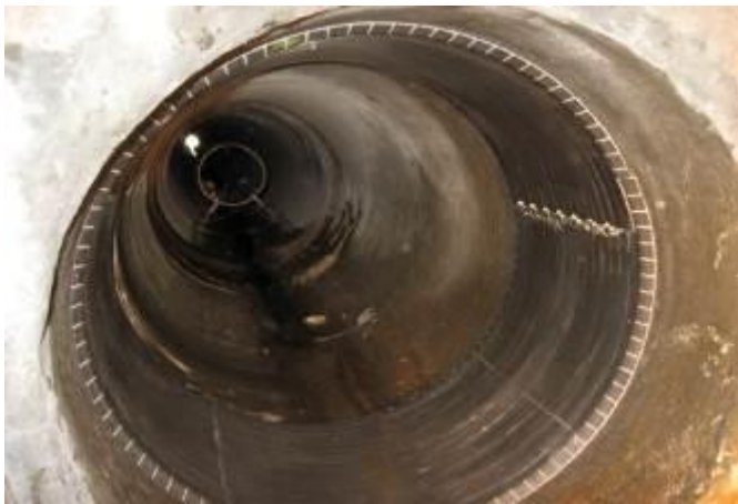
Photo 7: Link-Pipe Grouting Sleeve after installation over cracked conduit.
