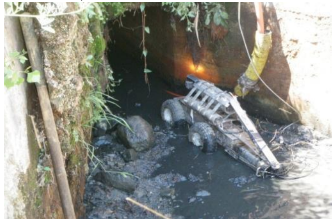
Photo 2: ROV entering a conduit for inspection.
