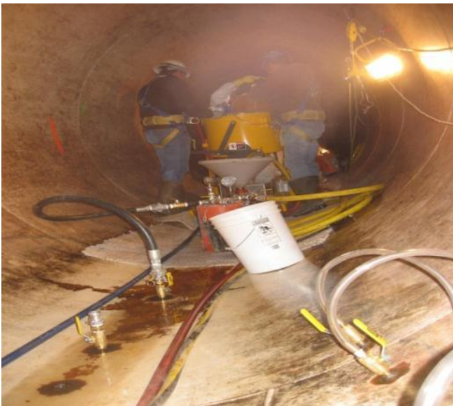
Photo 9: Injection grouting voided encasement behind steel liner.
