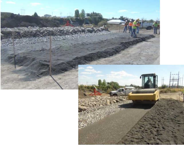
Photo 3. Test Pad for Granular Filter Materials
