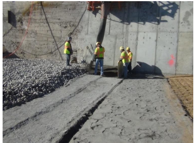
Photo 1. Placement of a 3-stage filter showing use of hand-held plywood shield to limit cross contamination.
