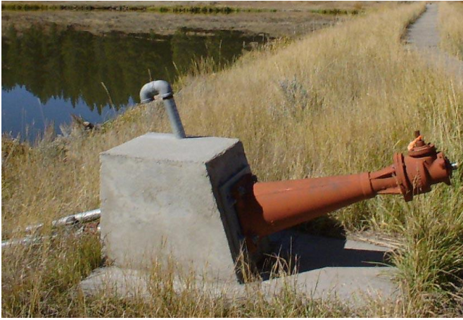
Figure 4: Typical outlet works air vent for a small dam
