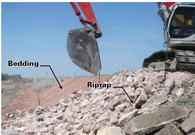
Figure 6: Placing riprap bedding and riprap on the upstream slope of a small dam in South Dakota.
