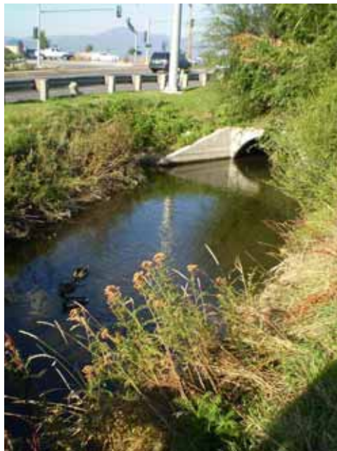
Culvert Under the Intersection of Mullan Road and Reserve Street
