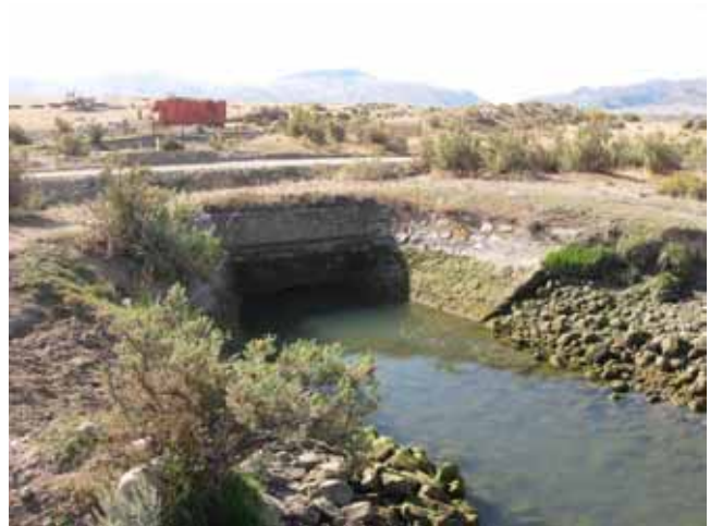
Anderson Siphon Exit
