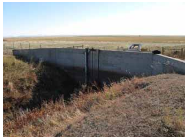
Headgate Structure within the Reservoir
