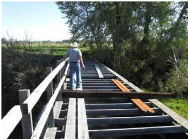
Ditch Operator Walking Across Structure
