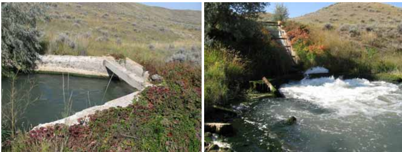
Two Leggins Canal Drop Structure North of Interstate
