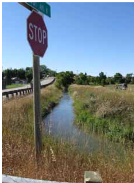
Ditch Running Parallel to Highway
