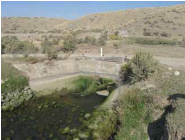
Anderson Siphon Entrance
