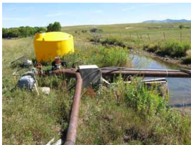
Pump Station – not operating due to low flows.
