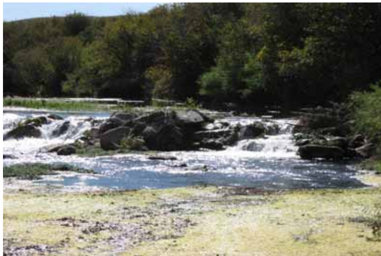
Kendall Ditch diversion dam - ditch channel is on the right side of the photo.
