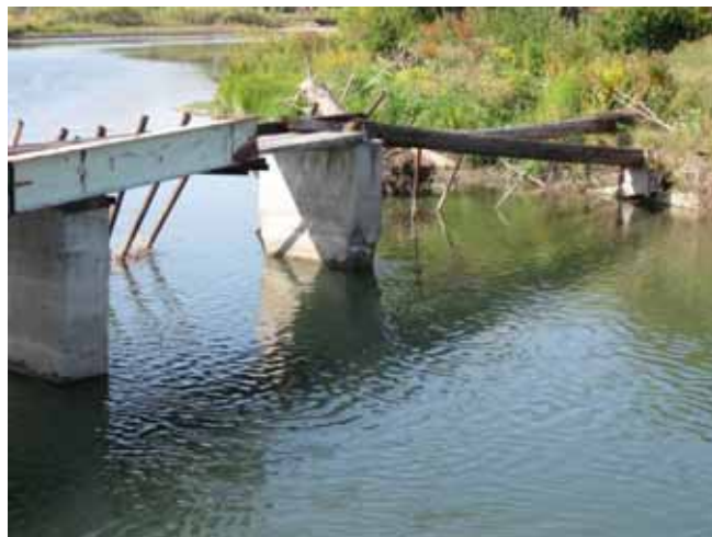
Trashrack in Front of Big Ditch Headgate
