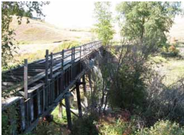
Wooden Flume – Spillway Visible in Center
