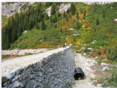
Mill Lake Dam as constructed by early irrigators in 1910.
